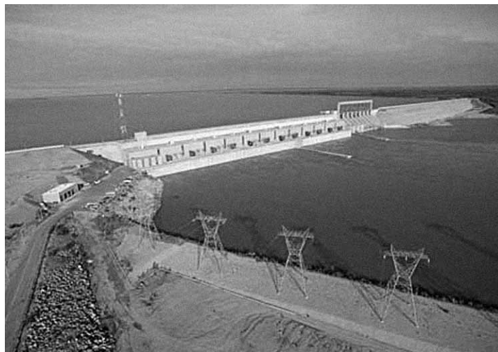
Kettle Plant (Source: Manitoba Hydro)
