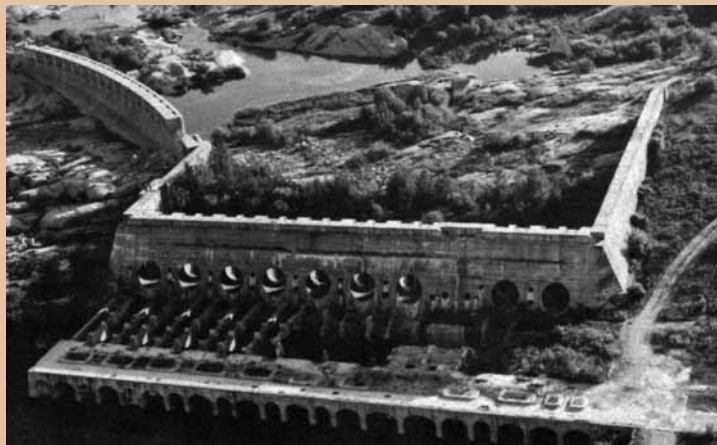
Pinawa Hydroelectric Power Project, 1906. Photo is from the IEEE Website: www.ieee.org
