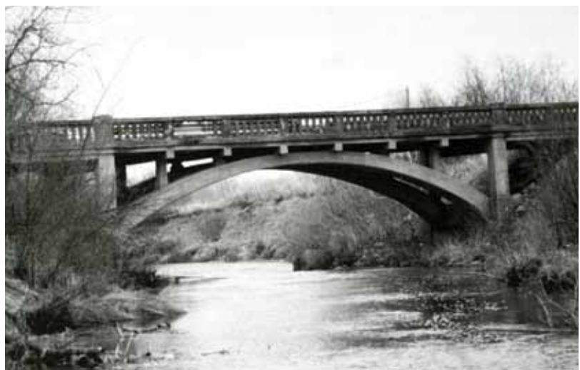
Whitemud River Bridge - 1916 - designed by M.A. Lyons Source: Archives of Manitoba
