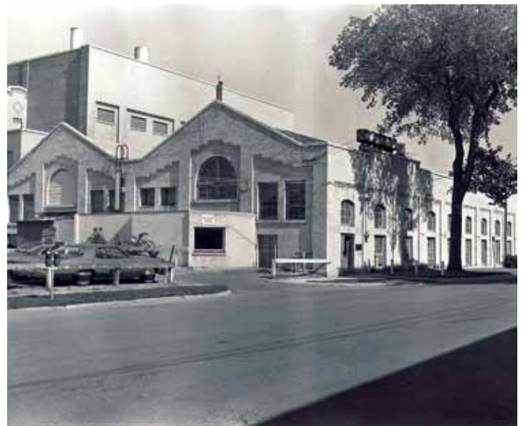
James Avenue High Pressure Pumping Station, ca. 1980 (City of Winnipeg, Planning Department)
