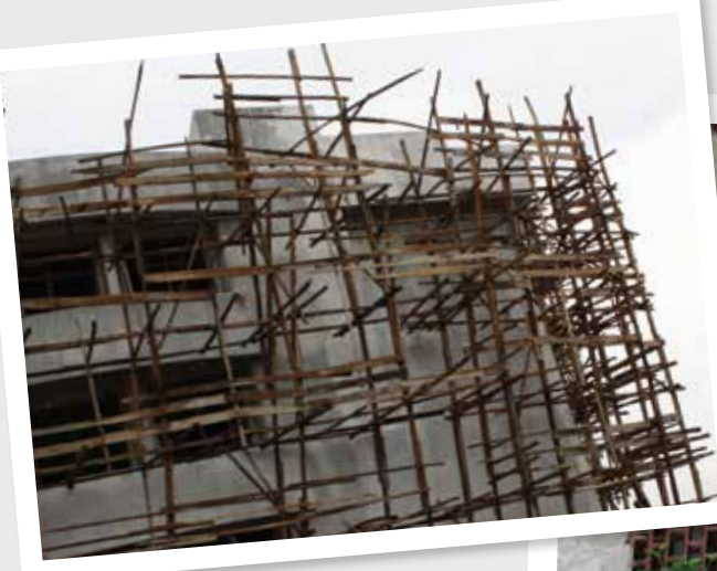
A construction site in Kigali, Rwanda. Jaimee Schmidt, P.Eng.
