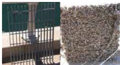
Figure 2: A trash rack from Parker Dam after 7 months in the Colorado River. (Source: Bureau of Reclamation)
