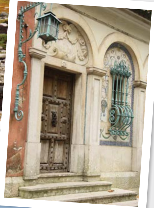
Elaborate doorway in Sintra, Portugal. Sintra is known for its many 19th-century Romantic architectural monuments, which has resulted in its classification as a UNESCO World Heritage Site. A. Kempam, P.Eng.
