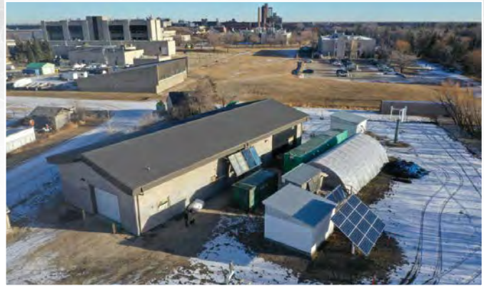
Sustainability-in-Action Facility (SiAF) located on the west edge of the Fort Garry campus.
